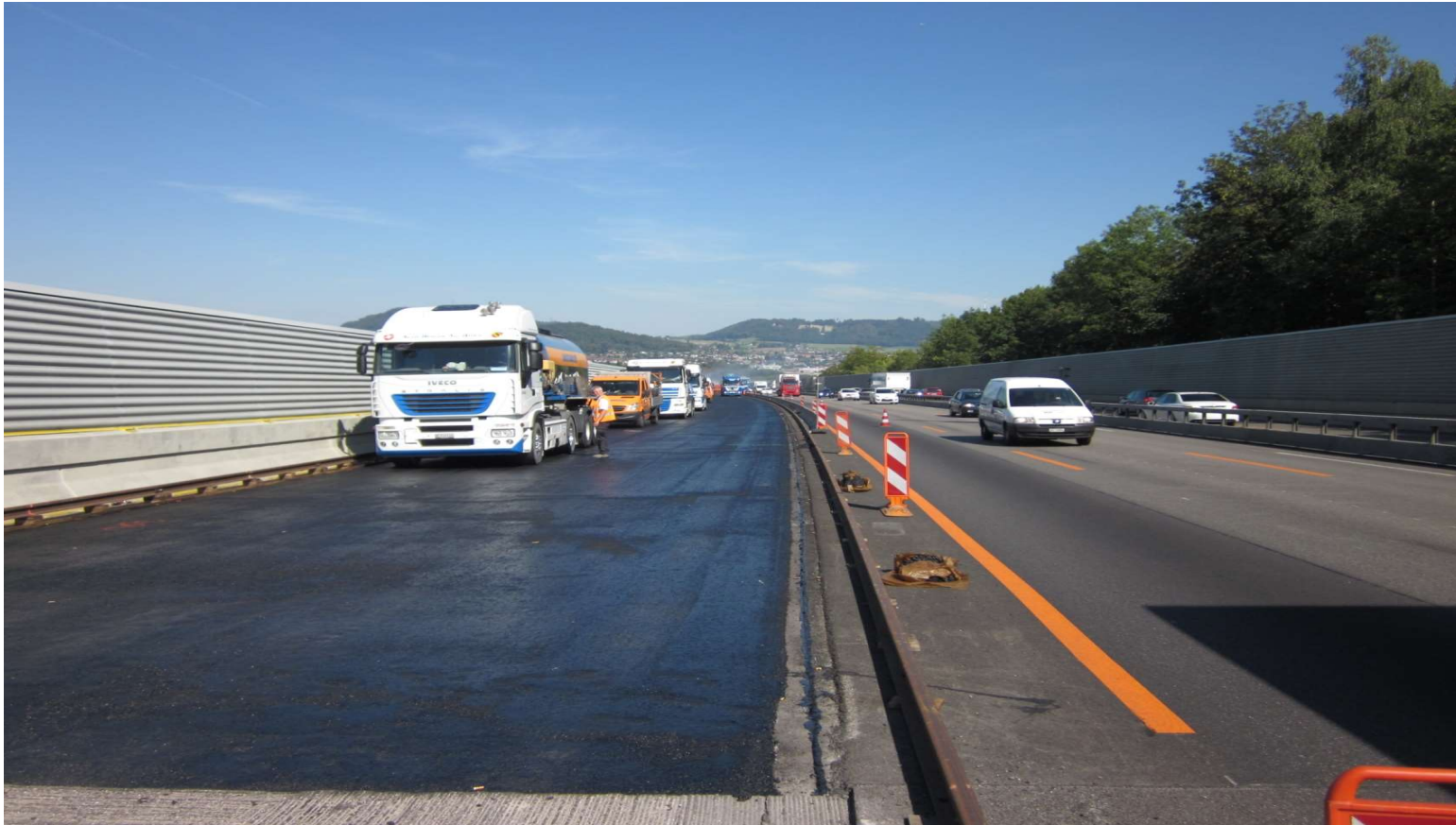
Mastic asphalt Switzerland
