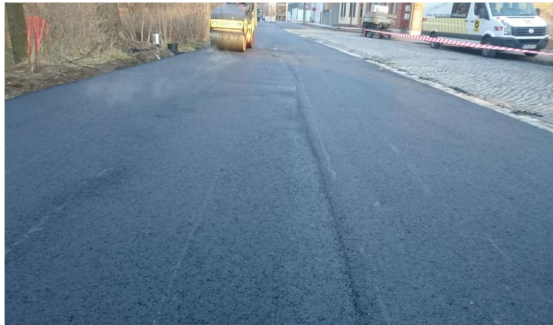
Test section in Greußen
